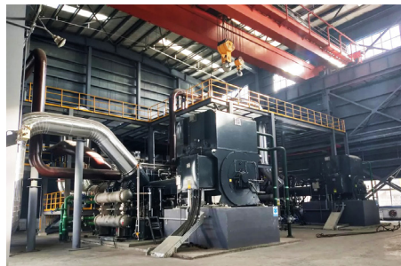
Left picture: Integrally-g geared refrigerant compressor (using a natural refrigerant). Right picture: A heat pump / mechanical vapor compressor with direct steam compression cycle applied in a chemical plant.
