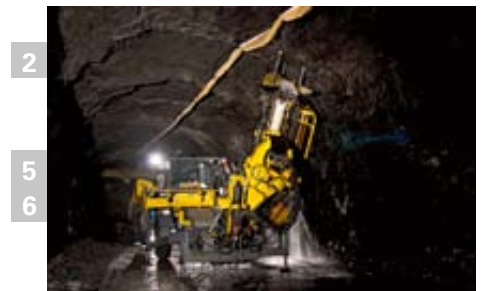
Simba for long-hole drilling
