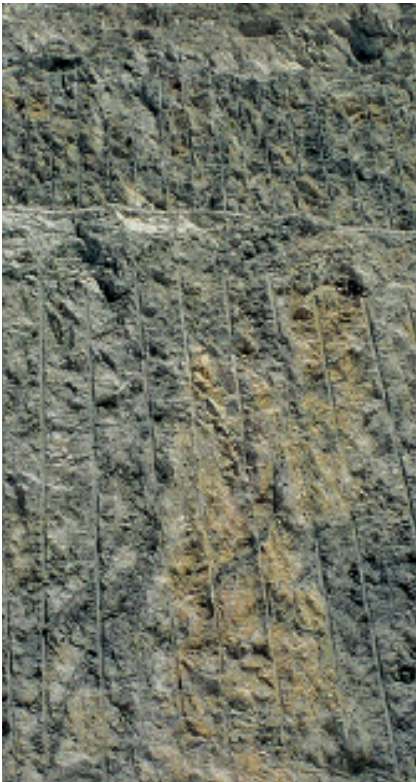
Figure 9. Near the pit wall more precise techniques are employed to minimize wall damage.
