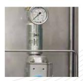
Very large bore emergency air actuated ball valves to isolate forecourt dispensers from high pressure gas flow sources
