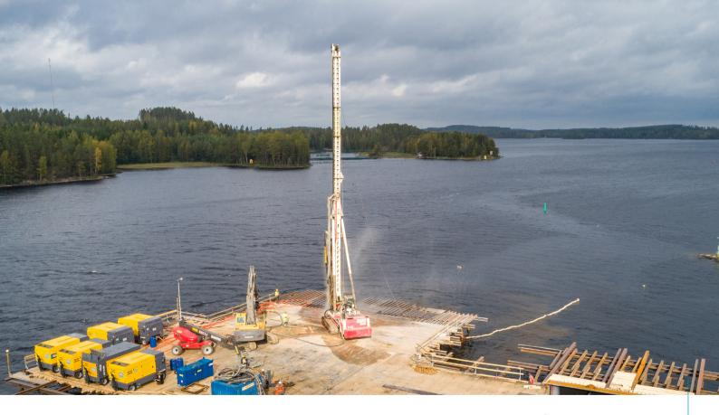
High-pressure air compressors producing 240 m³/minute of compressed air for the drilling of bridge pier piles in Finland. This high amount of air enabled more drilled meters with lower overall costs per meter.
