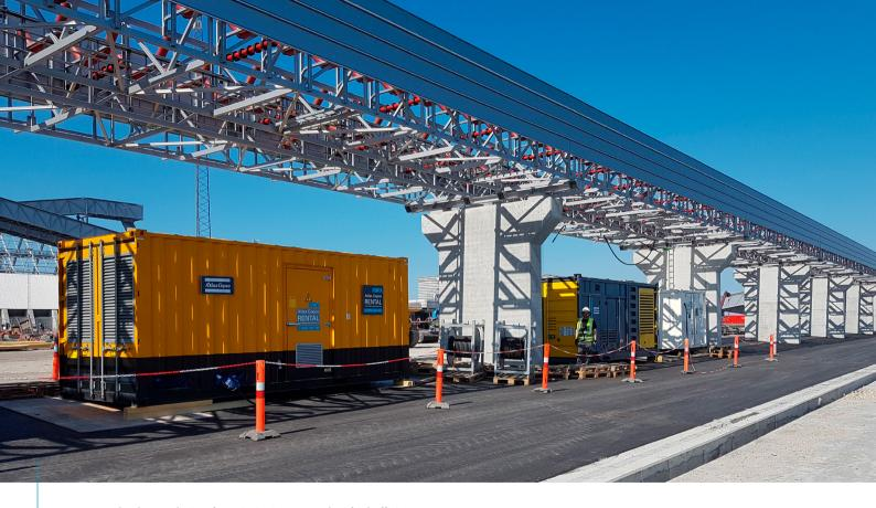
Temporary back-up solution for HOFOR in Denmark: a fuel efficient 1250-kVA diesel generator (400V) connected with a 2500-kVA transformer that converts and supplies cranes with 10 kV voltage.
