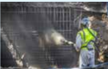
7 to 12 bar: Shotcrete applications
