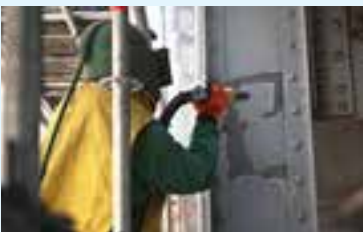
8.6 to 10 bar: Abrasive blasting
