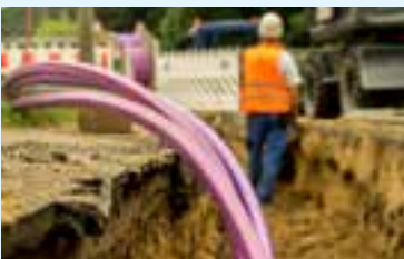
12 to 14 bar: Cable blowing and drilling
