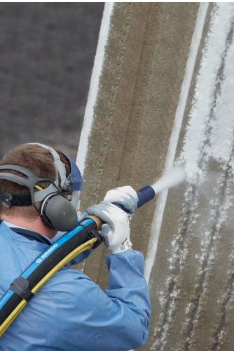
150 psi: Abrasive blasting
